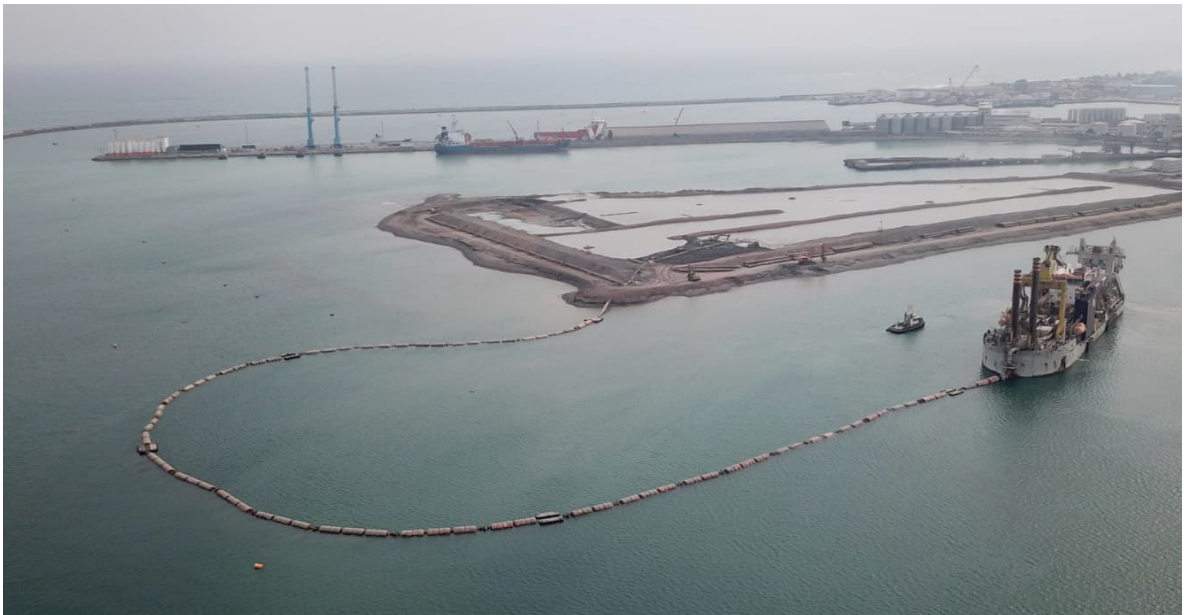
Figure 4-1: CSD, pipeline and reclamation area example
