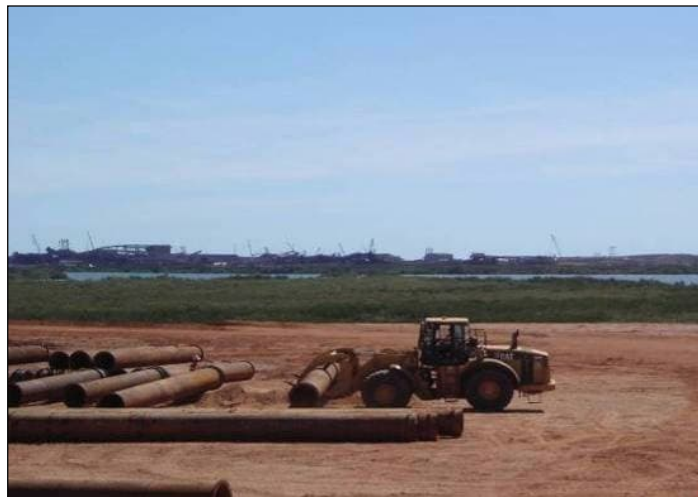
Figure 6-20: Wheel loader handling the shore pipes
