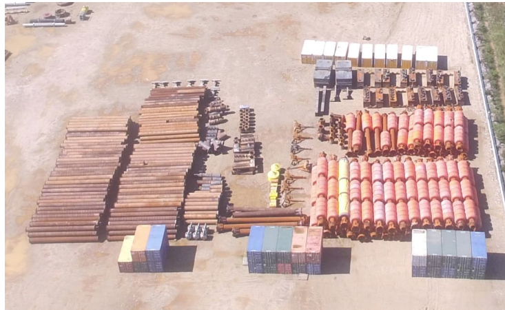
Figure 4-3: overview of equipment and pipes during mobilization
