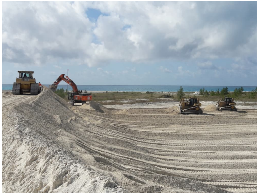
Figure 6-2: Construction of bunds with in-situ material
