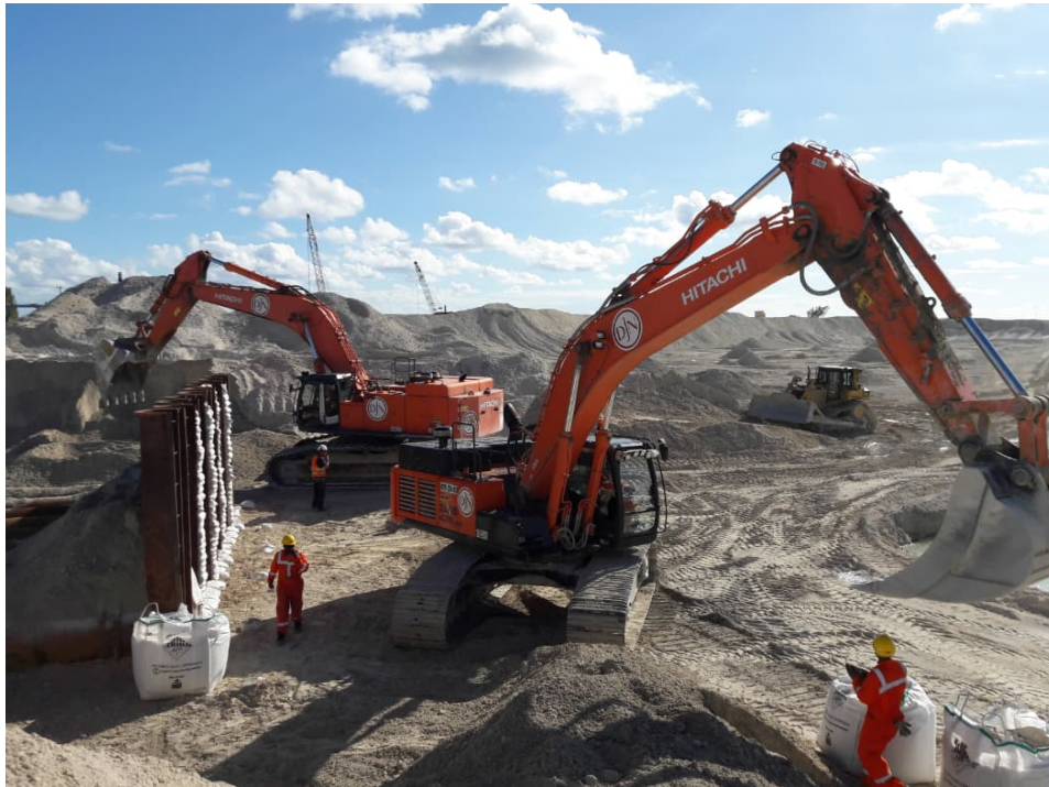
Figure 6-11: Installation of weirbox
