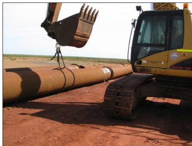
Figure 6-5: Lifting and positioning a shore pipe
