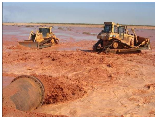
Figure 6-18: Outflow of material in discharge area, distributed by bulldozers
