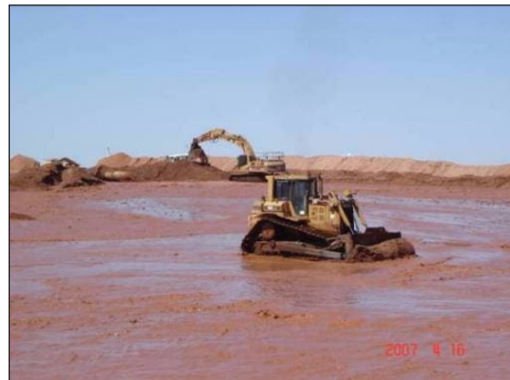
Figure 6-17: Bulldozer distributing the material in the discharge area
