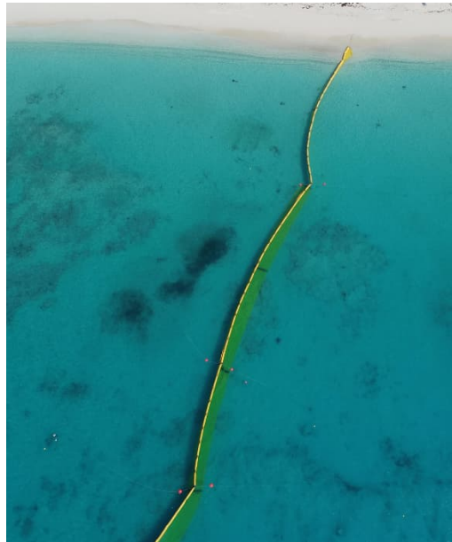
Figure 7-2: silt curtain along shoreline
