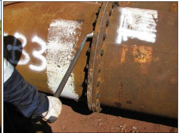
Figure 6-7: Tighten the bolts
