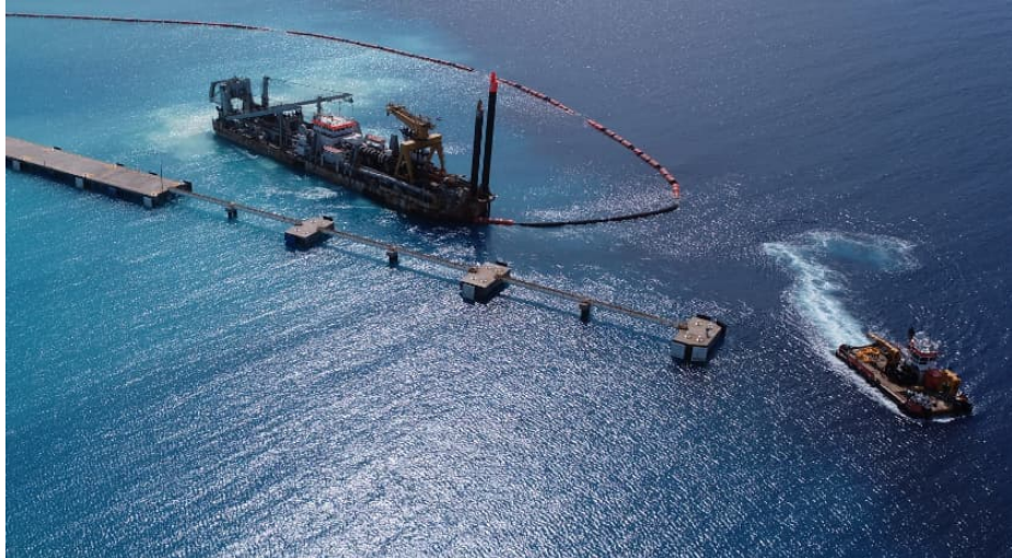
Figure 3-5: CSD and pipeline works
